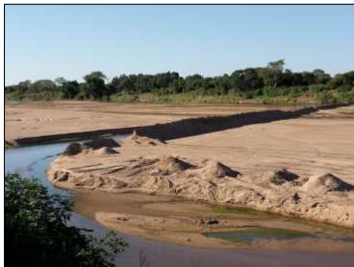
Figure 8: Artificial sand channels divert the flow of the Limpopo River towards the South African border (van Staden, 2015)
